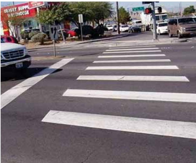
High-visibility crosswalks and vehicle stop bars improve the safety of pedestrians at crosswalks by making crosswalks more obvious to drivers. Image courtesy of safety.fhwa.dot.gov.
