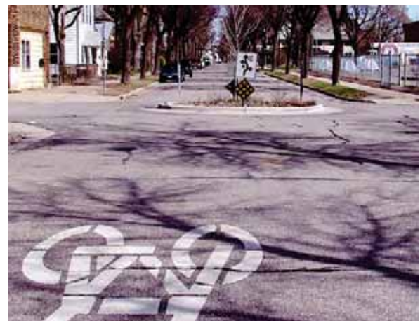
Traffic circles are present on the 5th Street NE bicycle boulevard where it intersects 15th Avenue NE and 17th Avenue NE, but needs better cues are needed for vehicles.
