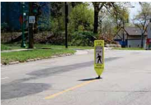
An in-pavement "Yield for Pedestrians" sign can greatly enhance motorist compliance with pedestrian crossings in low-speed neighborhood districts.
