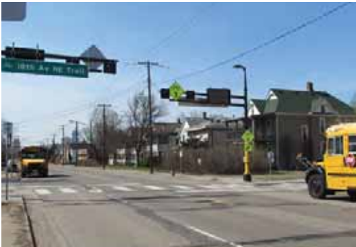
A no-parking zone should be enforced within a safe distance of the 18th Avenue NE Trail shared-use path crossing of University Avenue NE to provide better visibility for pedestrians and bicyclists using the trail. Here, two buses are seen parked close to the crossing.
