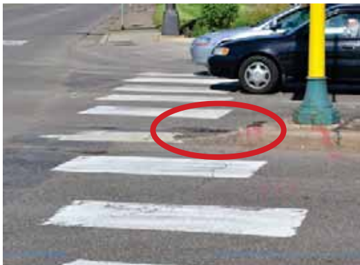
Median intrudes into the crosswalk and fails to offer protection to pedestrians crossing University Avenue along the northern edge of Broadway Street NE, near Sheridan Elementary School.
