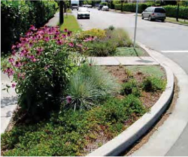
Curb extensions, or "bump outs," shorten street crossing distance and provide additional space for trees and landscaping. Image courtesy of commons.wikimedia.org.
